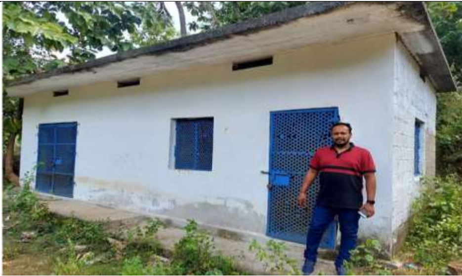
Figure 1: office building at a distance of 22m
